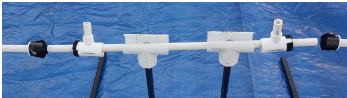
The new inter-array cable installed into two cradles.
