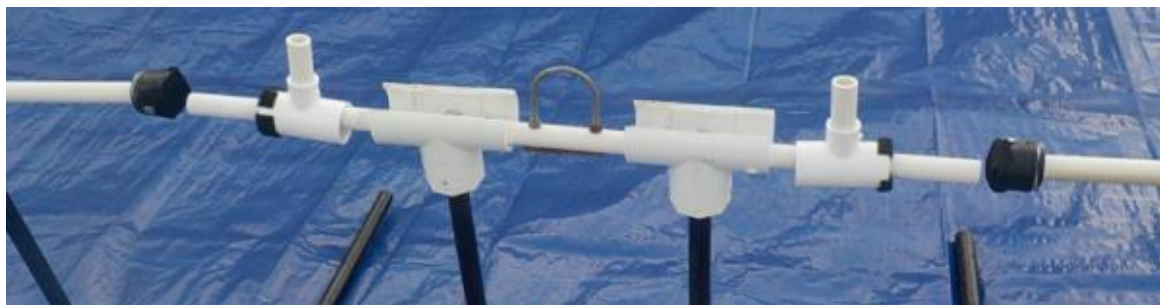
The new inter-array cable installed into two cradles.
