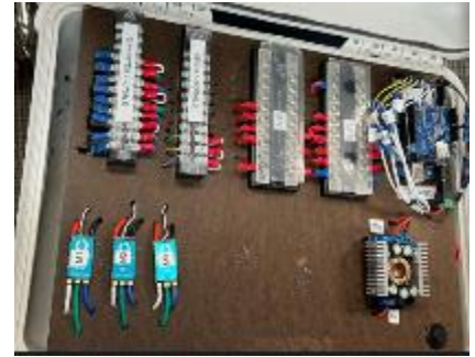
Figure 5: Kraken surface control, showing neatness and attention to workmanship.
