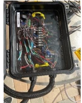
Figure 12: Inside view of the control box.
