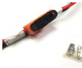
Picture 23 - 25A fuse installed on the power cable
