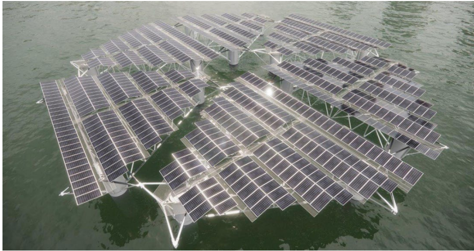
SolarDuck floating panel solar arrays ( SolarDuck and Partners to Build and Test Offshore Floating Solar Platform ‘Merganser’ | Energy | News (oceannews.com) )
