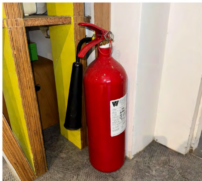
Figure 18: The fire extinguisher below 3D printers
