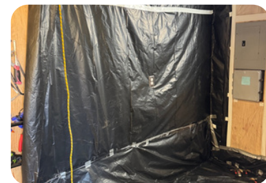
Figure 42: Clean room while being built - Photo by Robert McIntosh
