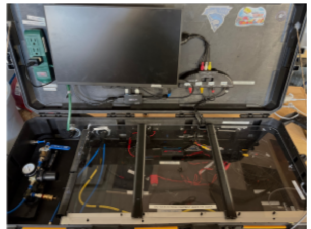
Figure 9: Siku control box - taken by James Penney
