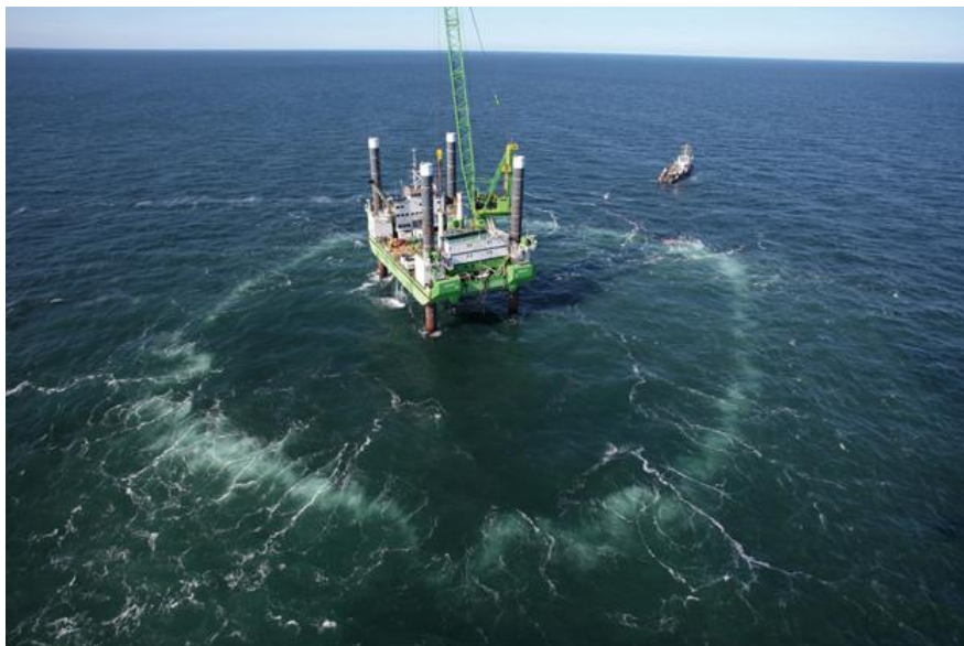
A bubble curtain around the area during installation of an offshore wind farm in Germany. Bubble curtain - Wikipedia
