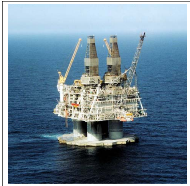
Hibernia oil production platform
