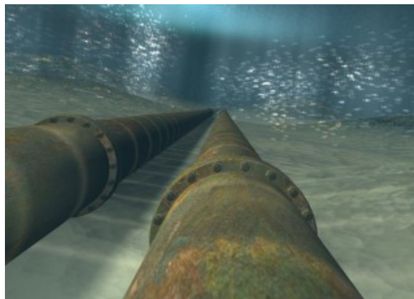
Corroded subsea pipeline ( http://subseaworldnews.com/2014/04/01/baosteel-yantai-delivers-subsea-steel-pipes-for-bohai-oilfield/ )
