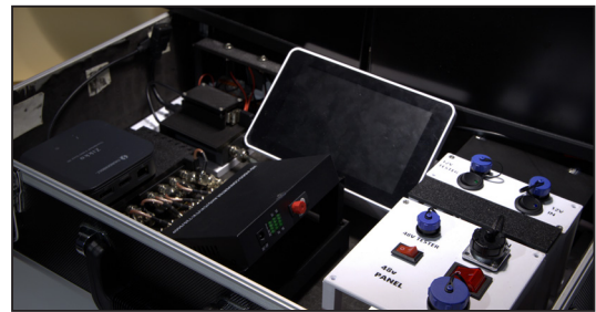
Figure 32. Control box electronics
