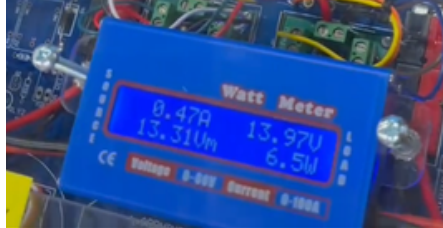
Fig. 9. Control Box screen displaying real time power consumption
