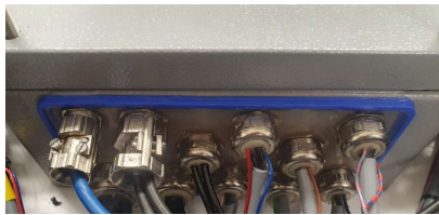
Figure 12: epoxy resined frame
