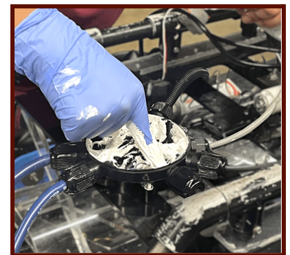
Figure 17: Sealing the Junction Box Photo Credit: Eric Fernandez
