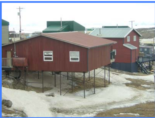
Figure 15. House on support beams in Iqaluit.
