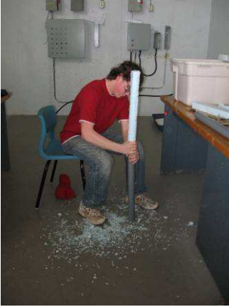
Figure 12: Alex fitting foam into a pontoon
