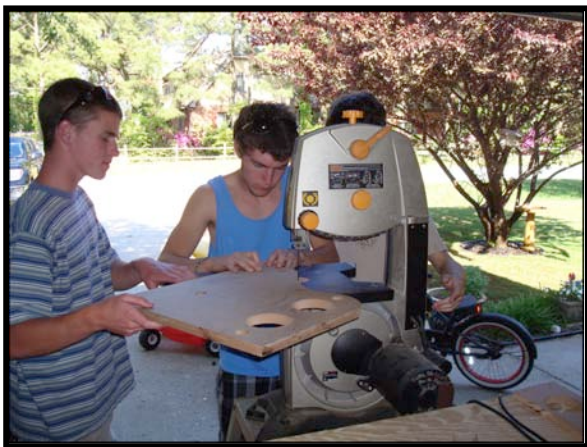
Figure 6: Cutting the template for our framework out of MDF. (Photo: Thomas)
