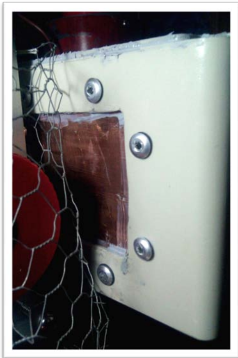
Figure 5: Copper plate water cooling
