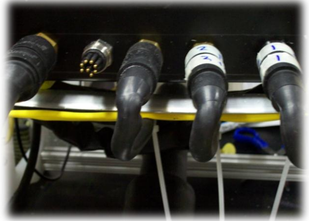
Figure 8 – SubConn bulkhead connectors drilled into dry housing
