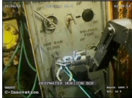
Figure 14 - Still capture of a video feed from one of the ROVs working on the well
