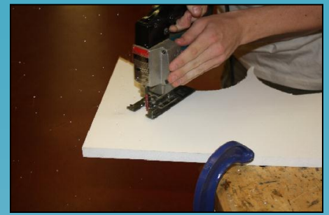
Figure 35- A team member cutting through the sheet PVC
