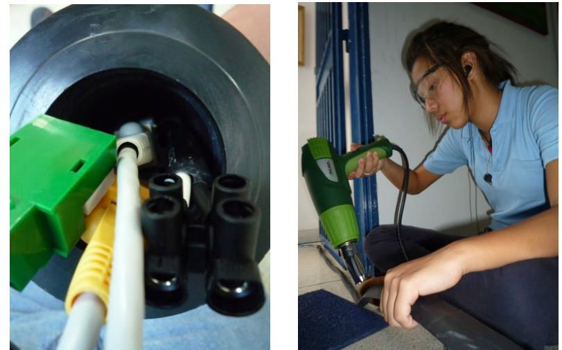
Figure 22. Left, inside view of the decoupling system. Right, 25 mm heat shrink applied to the tether. R.M.
