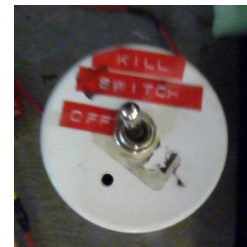
Fig 1.11 Control Panel kill switch
