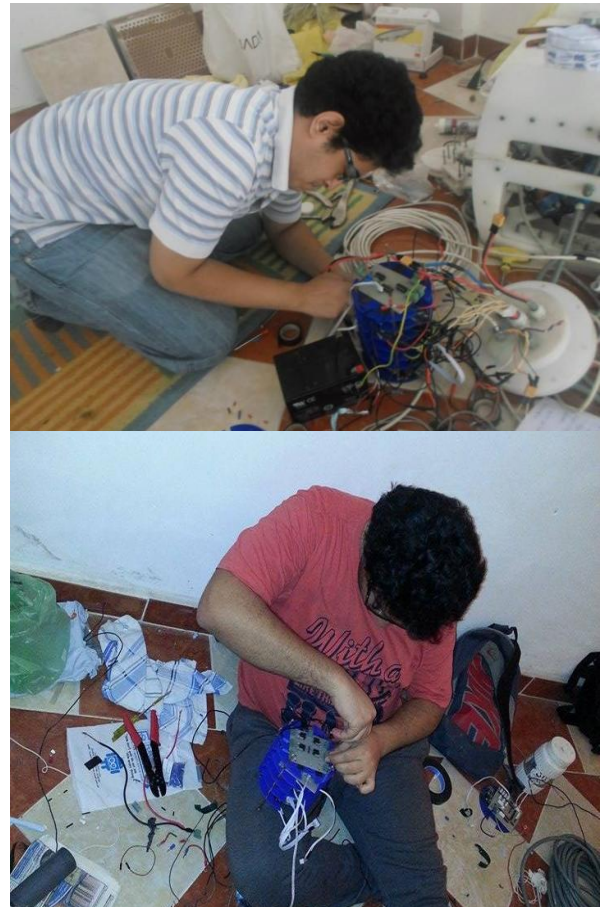
FIGURE 29 - SIEF AND AHMED FAROUK TROUBLESHOOTING WIRING DEFECTS
