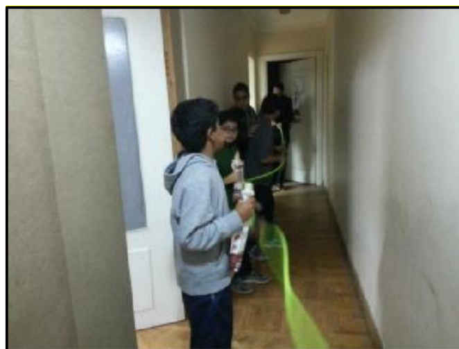
Figure 44 Sea Pearl team members casing the wires.
