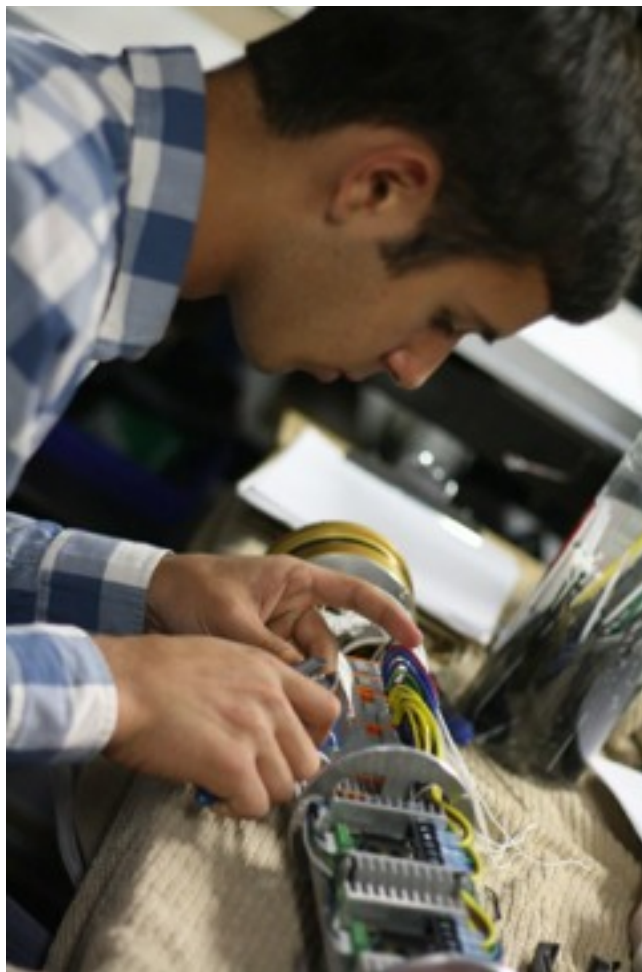
Image 16: Team member wiring onboard controls on housing skeleton.
