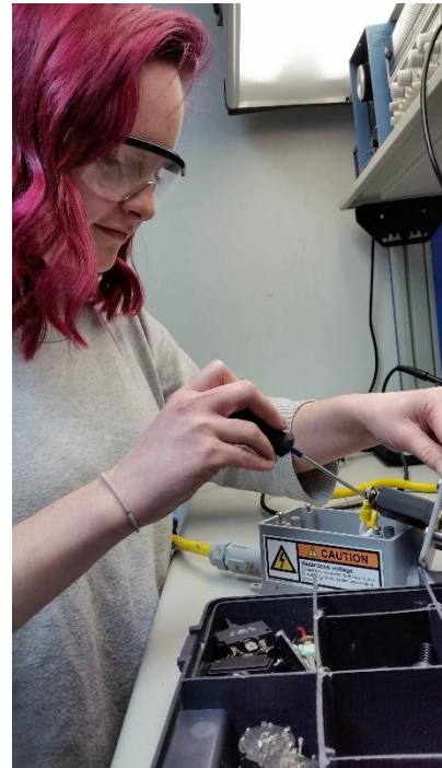
Figure 17: Racheal installing a new topsides circuit breaker
