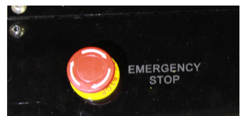
Figure27: Emergency stop button for troubleshooting
