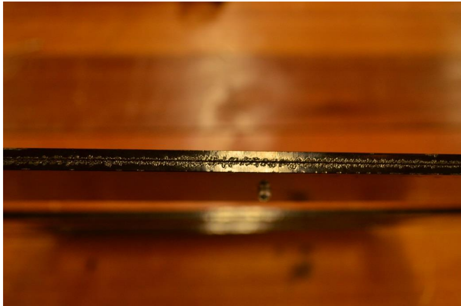
Side panel consisting of two layers of polycarbonate bolted together Photo by Alexina Haefner
