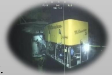
Figure 4: ROV repairing a wellhead cap -Associated Press
