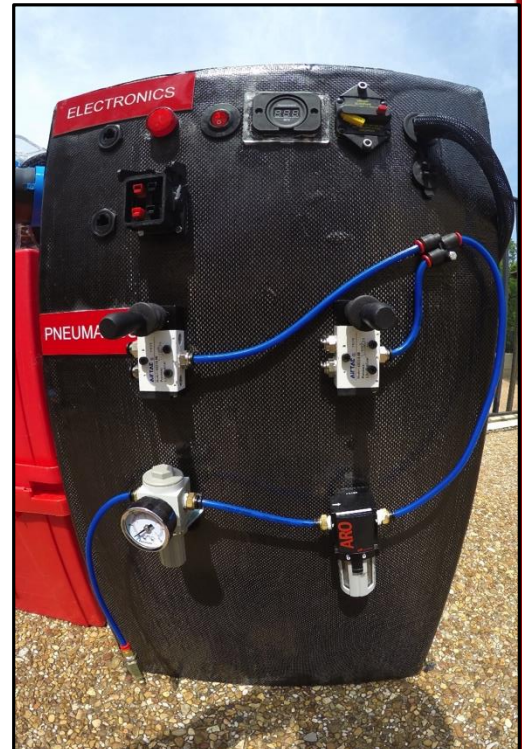
Figure 15: Pnuematic Controls with pressure regulators -Mack Van Wagnen
