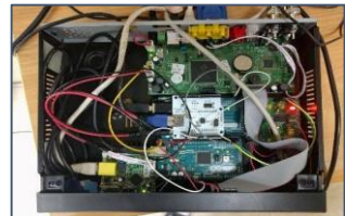
Figure 17 - DVR casing after adding station boards inside
