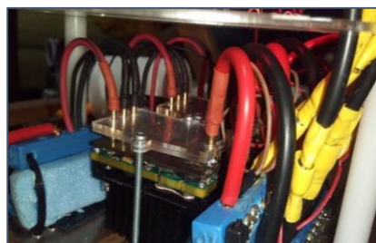
Figure 20 - DC Converters fixation and wiring at the lower tray
