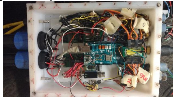
Figure 10- Internal electronic components
