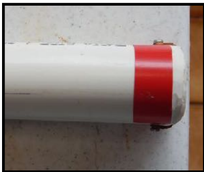
Figure 15: Red electrical tape on the sediment collector to indicate a sharp edge. (Credit: L. Adcock)
