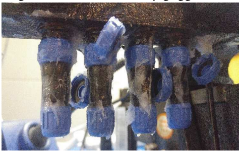
Figure 33 Plugs connected to the sockets covered with petroleum jelly while casting epoxy (By: Joshua Ho)
