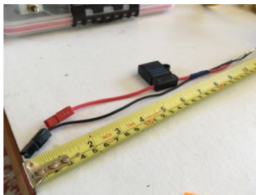
Bottom inside of our control box.
