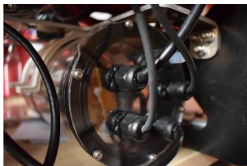
Figure 7 Cable glands going into control boxes. Captured by Marwan.
