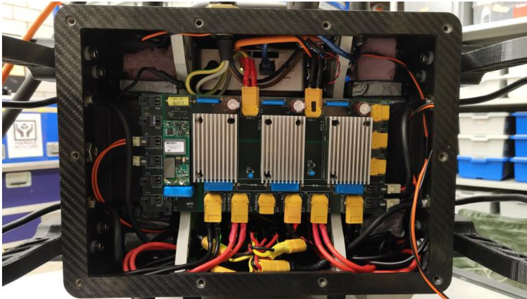
Figure 14: Placement of the DC/DC converter PCB inside the ROV.
