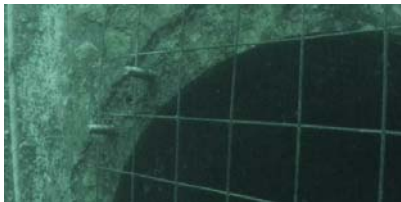
ROV image of an intake gate.
