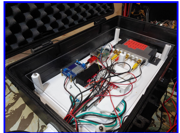
Figure 3.0 Inside view of the EHC
