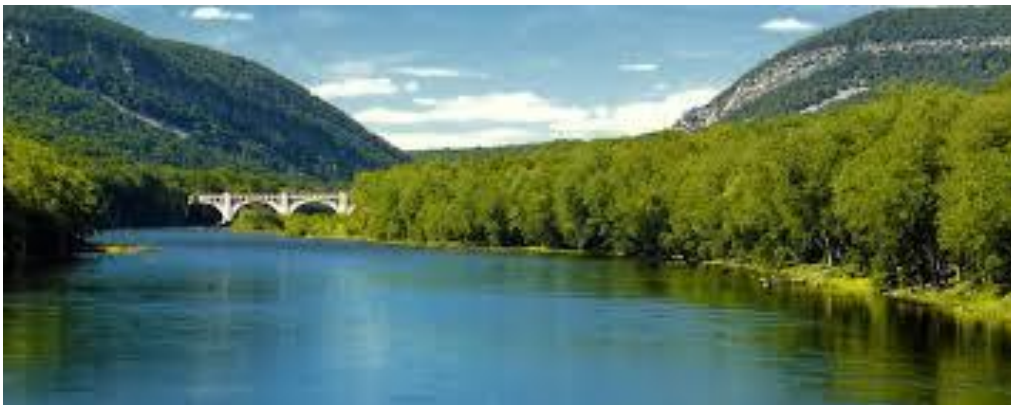
Photo 3: Delaware River Credit: American Rivers 2
